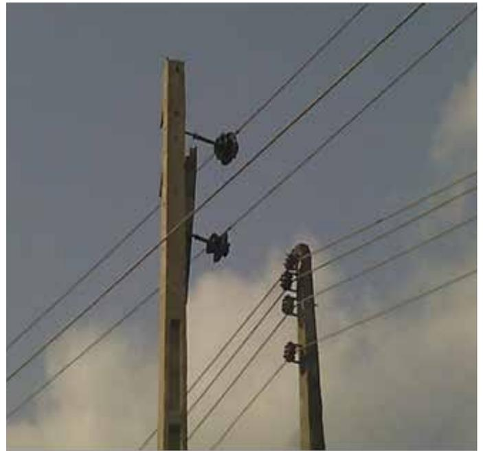
Figure 4 Broken cross poles
