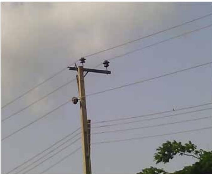
Figure 3 Broken cross poles
